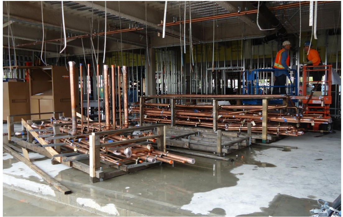
Mechanical systems off-site racking – Mesa College Math & Science Building
