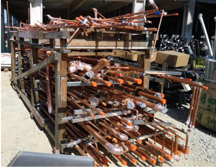
Mechanical systems off-site racking – Mesa College Math & Science Building
